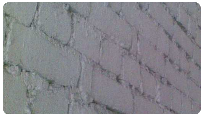
Fig. 2 Dust is captured in open grouting.
